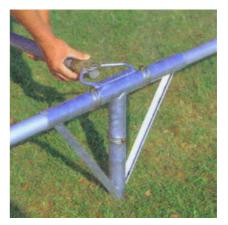
The next step is to connect all the struts to the crowns, this can take a bit pulling and pushing as it is at this stage any unevenness in the ground or the corners not being square will become apparent.
