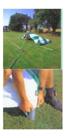
Now place a leg next to each corner and T section. One person then prepares to slot the legs into place whilst the rest of the team lift one side of the marquee.
